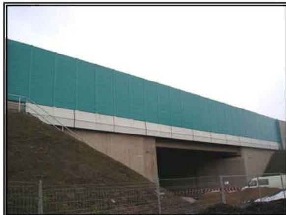
The single-sided highly absorptive noise protection panel consisting of sea-water resistant aluminium is powder coated outside. It is made of structural bearing roll-formed and folded lateral aluminium parts and vertically stabilizing end caps. It has been designed for installation in posts of the HE\_160 series.
